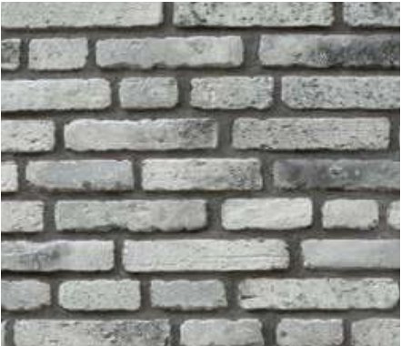
BQ-006 Grouting GM-01
