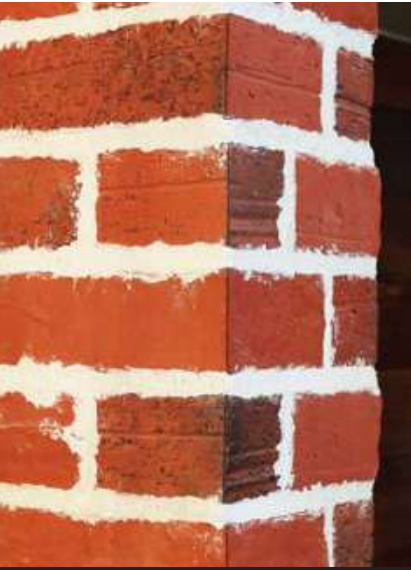
45° Cut and Join Technique
