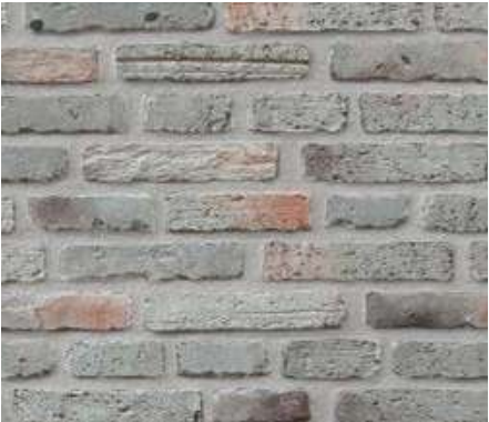
BQ-004 Grouting GM-11
